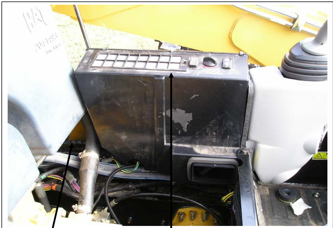
A/c lines and relay control wire.
